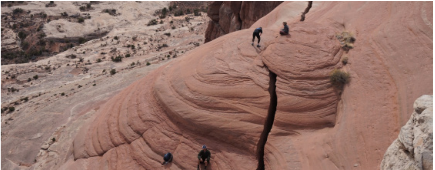
Part of a 500 meter-long crack in the Jurassic Entrada Sandstone delineating a toppling mode rock slope instability. The fracture is site instrumented with a UofU seismometer and a crackmeter. AEG (Association of Engineering Geologists) GeoHazard field trip, March 2020
