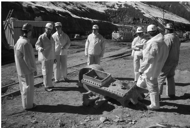
Tanner Ridge Tunnel portal at Diamond Fork, UT
