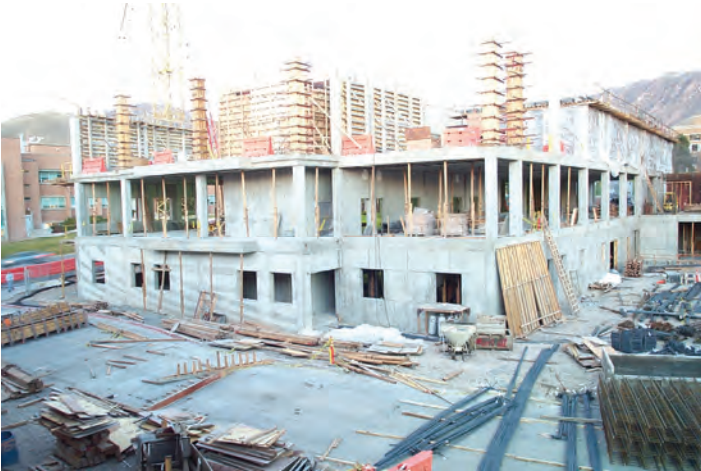
2. The walls begin to rise. See the cross-bedding in the foundation?
