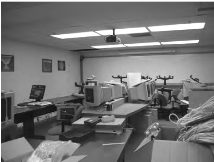
Computer lab during renovation.
